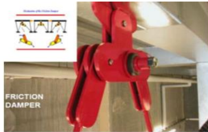
Figure 1: Using rotational friction dampers in retrofitting.
